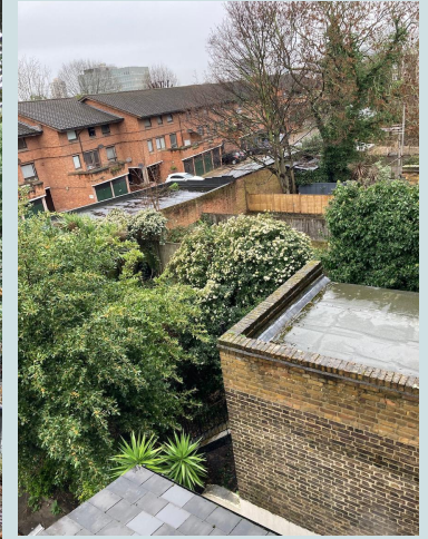
adjoining back gardens
